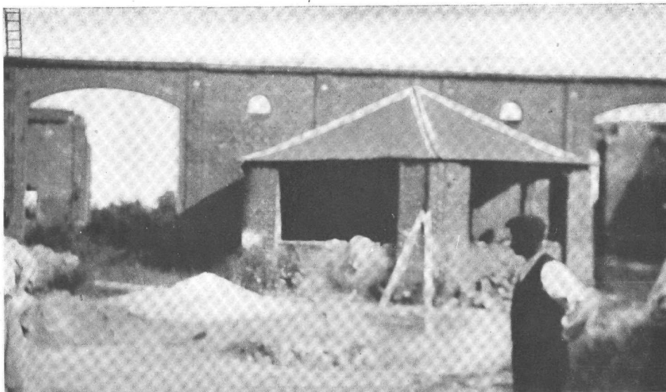
View of Imberfayt Farm, taken during the summer of 1920
