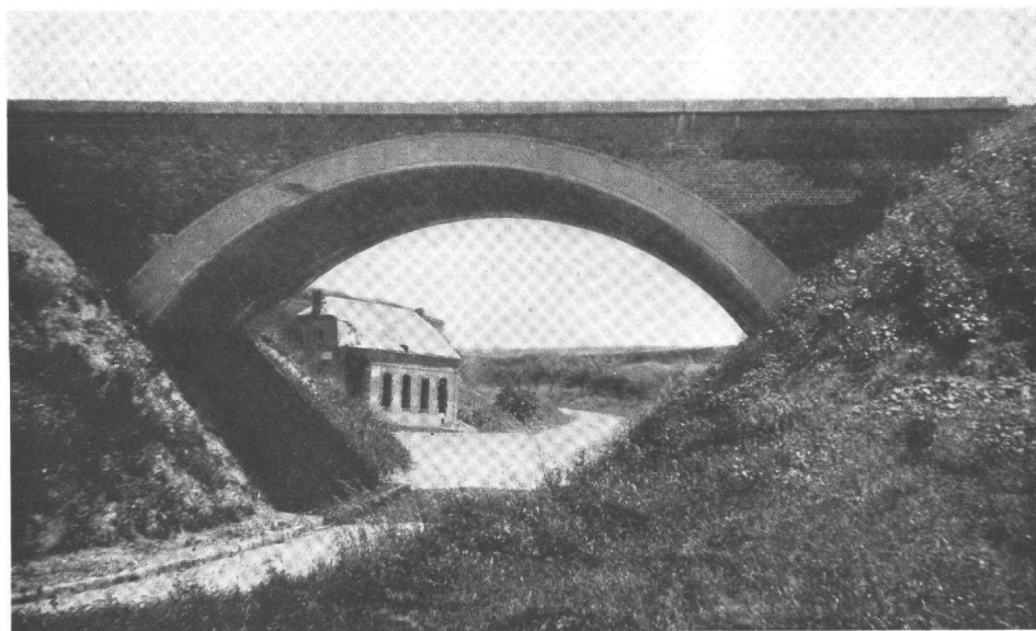
Permanent bridge built across Le Selle River at St. Souplet after the Armistice. Picture taken during the summer of 1920
