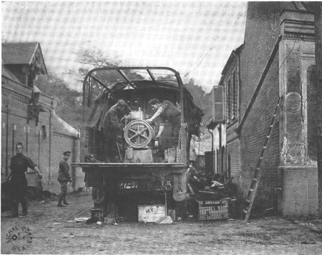
27th Division National Guard mobile electric light plant, Corbie, France
