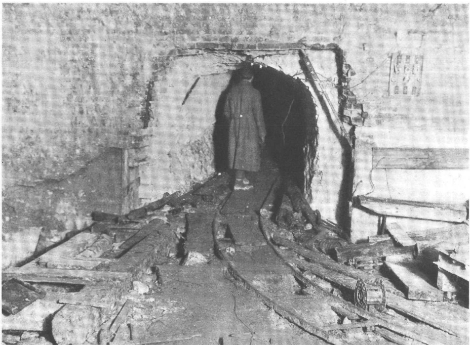
One of the many passages cut from the tunnel to the trenches
