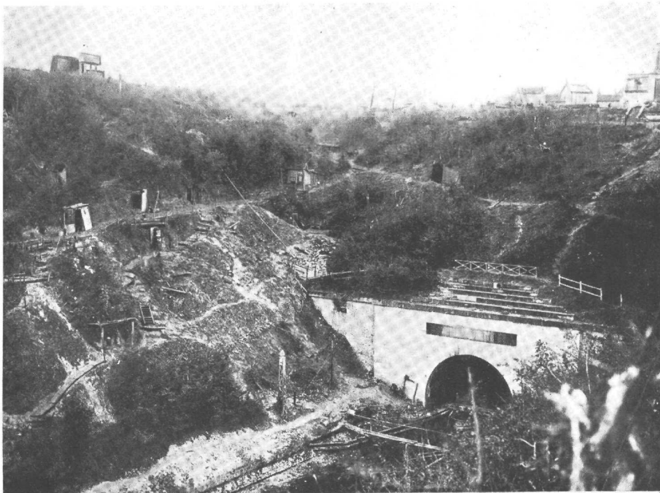
View of St. Quentin Canal Tunnel
