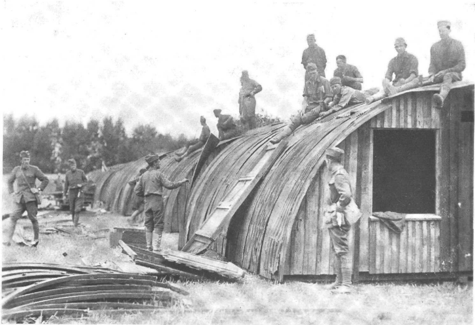
102d Engineers finishing "Nissen" huts at St. Laurent, for use of Headquarters 27th Division. Due to changes in orders, however, Division Headquarters did not occupy these huts
