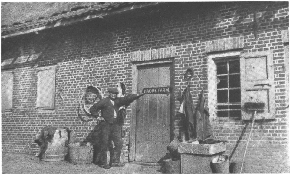
A close-up view of one of the buildings at Hague Farm. Photo taken summer of 1920
