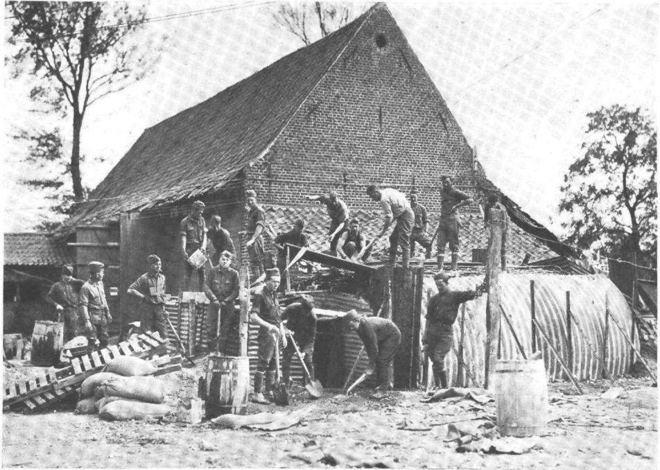
102d Engineer Train constructing dugout for telephone and telegraph for the 105th Infantry Headquarters during the Battle of Vierstraat Ridge
