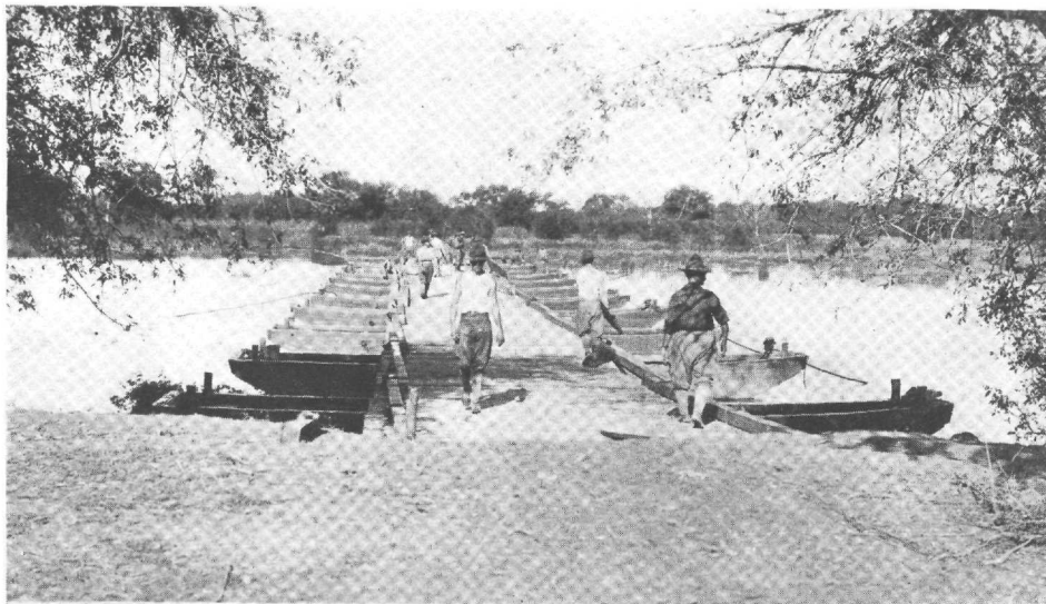
Heavy pontoon bridge erected by the 22d N. Y. Engineers west of Mission, Texas
