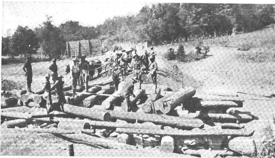
"Snake Road" undergoing repair. View of bridge No. 1 under construction
