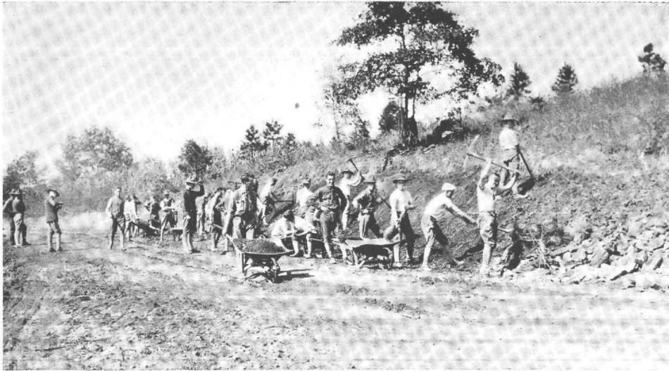
Widening the "Snake Road" to fifteen feet
