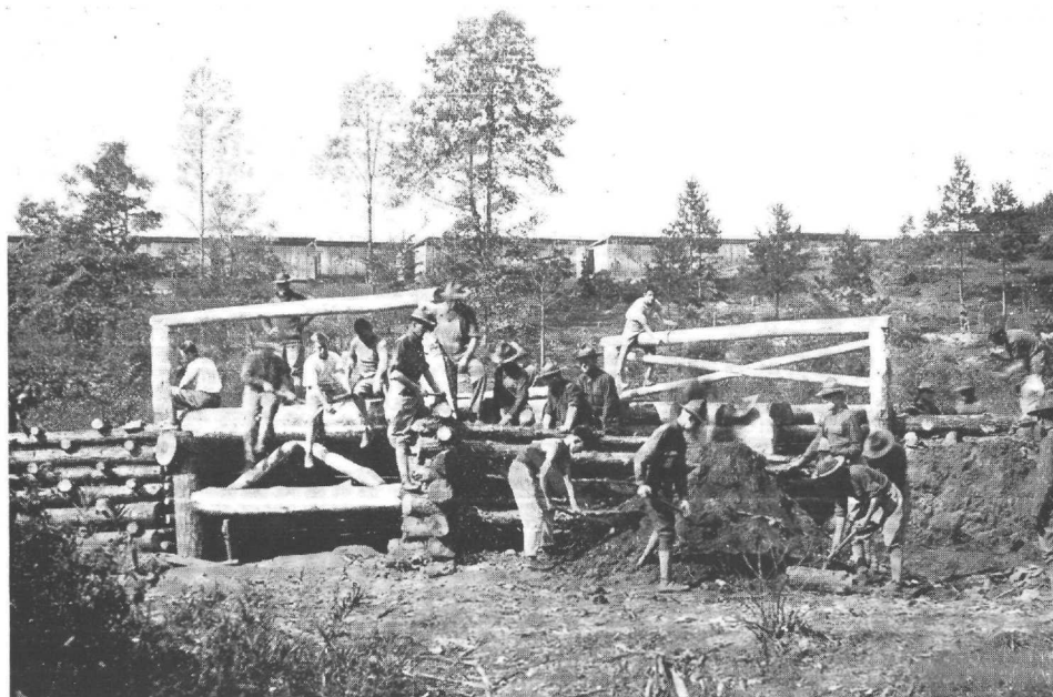
102d Engineers repairing the "Snake Road"
