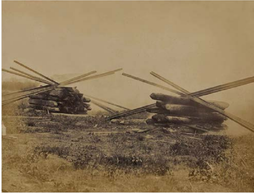
Military railroad operations in northern Virginia – Iron rails were twisted by positioning them over piles of wooden railroad ties which were then burned (ca. 1862-'63)
