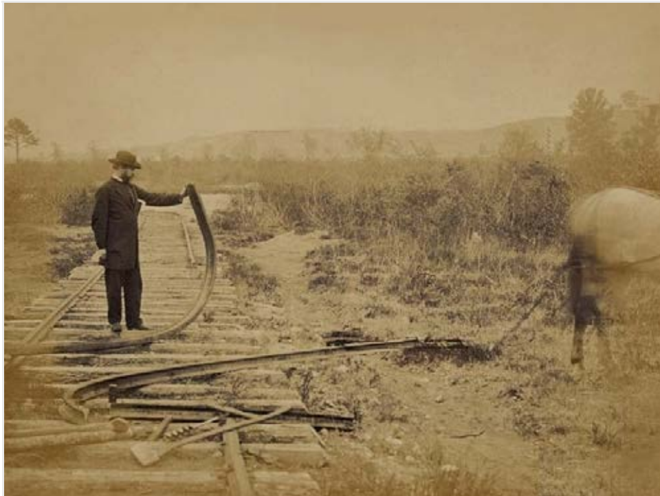
Military railroad operations in northern Virginia – Iron rails were twisted by positioning them over piles of wooden railroad ties which were then burned (ca. 1862-'63)
