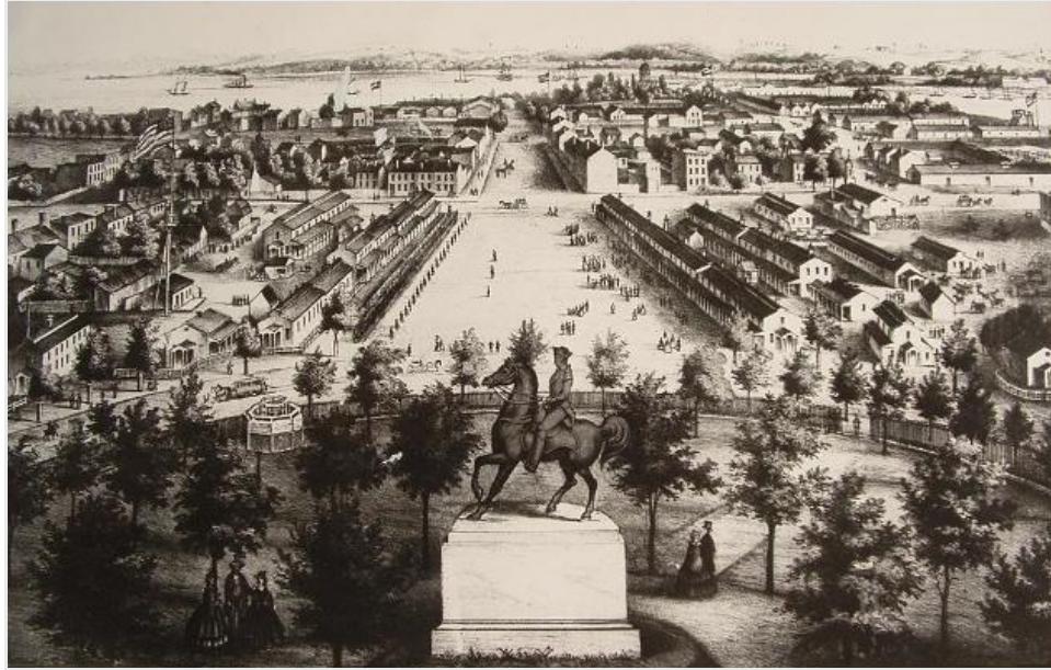
Washington Circle, with Camp Fry to the south
