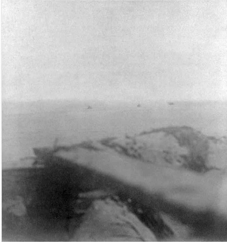
View from the parapet of Fort Sumter showing the U.S. Monitors "Weehawken," "Montauk," and "Passaic" firing on Fort Moultrie (September 8, 1863)
