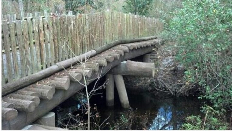
Bridge at McGirt's Creek, Camp Milton Historic Preserve, Florida
