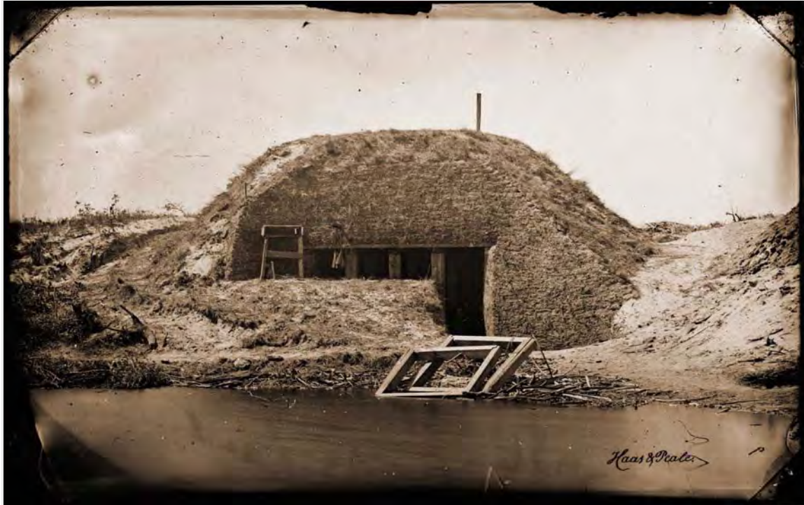
Bomb-proof for telegraph operator in trenches, Morris Island, South Carolina (ca. 1863)
