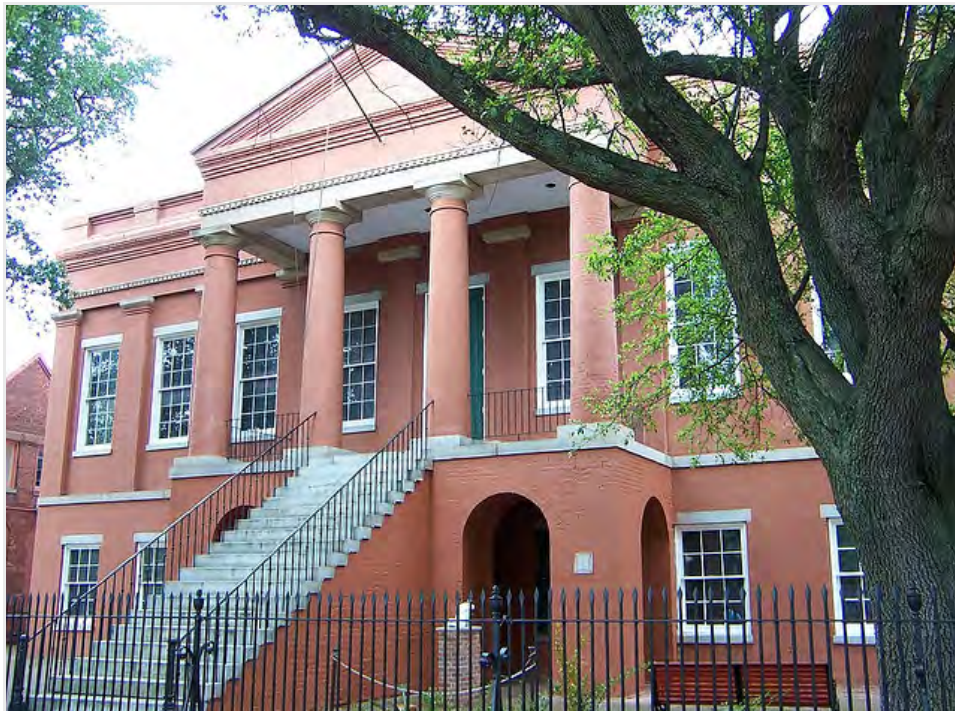
Portsmouth Courthouse, now the Portsmouth Art & Cultural Center
