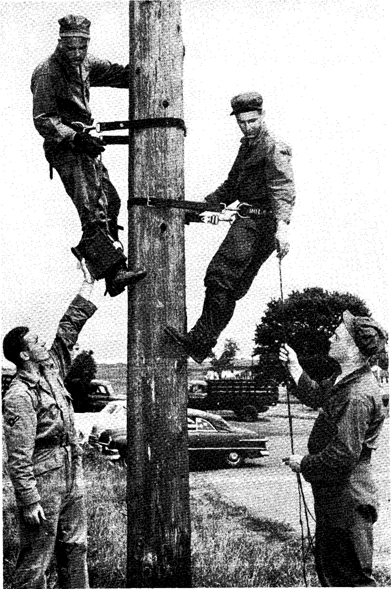
Linemen of the 107th Communications Squadron, N.Y.A.N.G., are shown installing a communications system at Spaatz Field, Pa., where the unit and other squadrons of the 107th Fighter Interceptor Wing, N.Y.A.N.G., were in summer training in 1953. Shown, clockwise, are Airman 3/c Richard Killian of 15 Collingwood Ave., Buffalo; Basic Airman Thomas Neelan of 316 Odgen Road, Tonawanda; Airman 3/c Donald Harder of River Road, Tonawanda, and Sgt. Eugene Donahue, the wire chief, of 506 Delaware Ave., Buffalo
