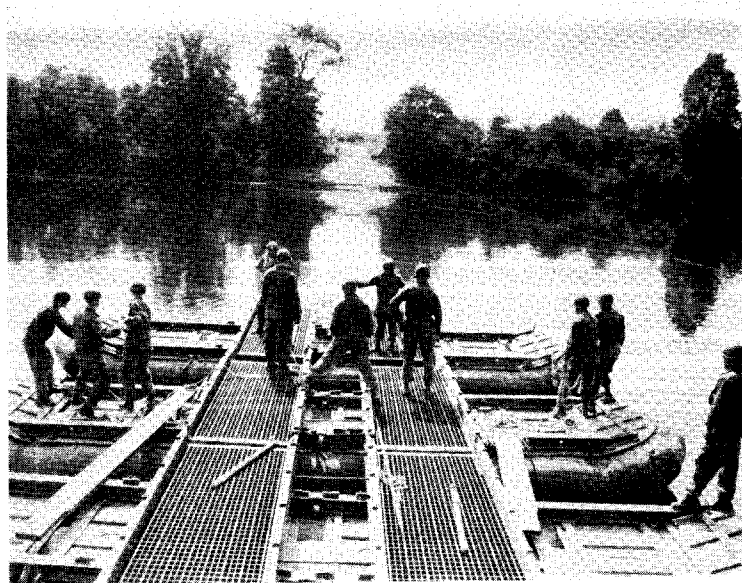
40 ton treadway bridge, issued to divisional engineer battalions
