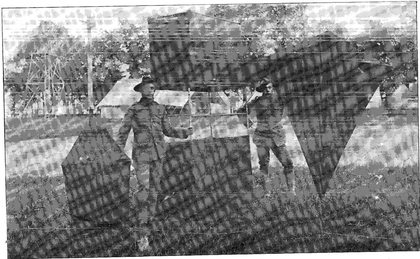
KITES BUILT BY THE FIRST COMPANY, SIGNAL CORPS, FOR CARRYING INTERNATIONAL CODE SIGNAL FLAGS AND THE ANTENNAE FOR WIRELESS TELEGRAPHY, CAMP OF INSTRUCTION, PEKSKILL, N. Y., JUNE, 1907.
