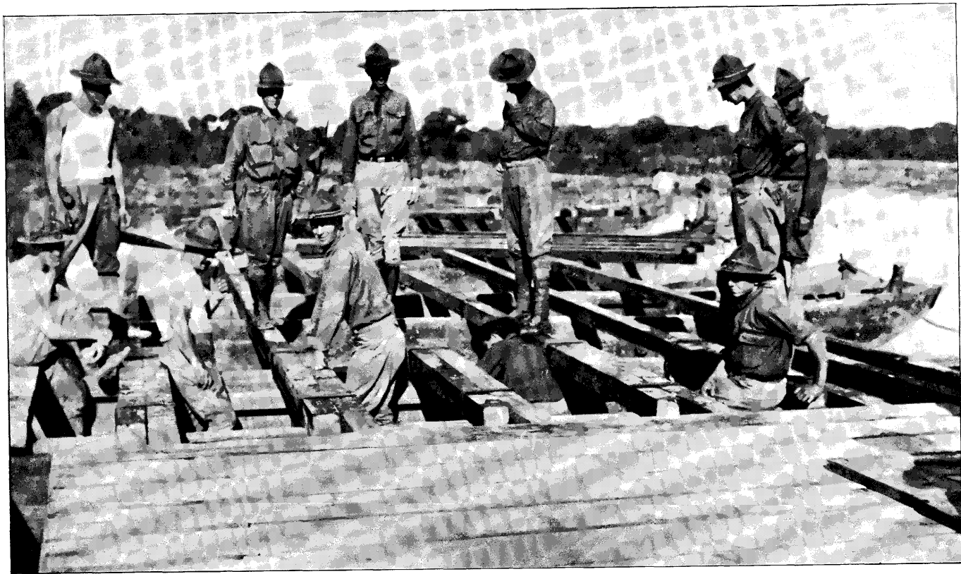
22D NEW YORK ENGINEERS CONSTRUCTING A PONTON BRIDGE AT PEÑITAS, TEXAS
