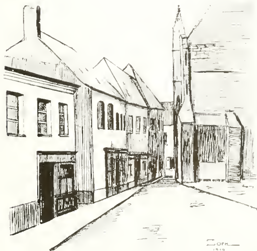
This Street in Rue Should be Familiar to Most of Us
