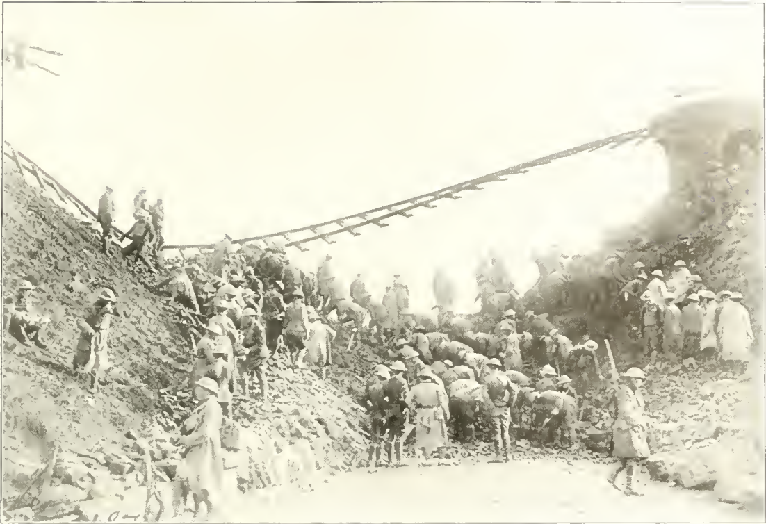
102d ENGINEERS AT ST. SOUPLET BRIDGE
