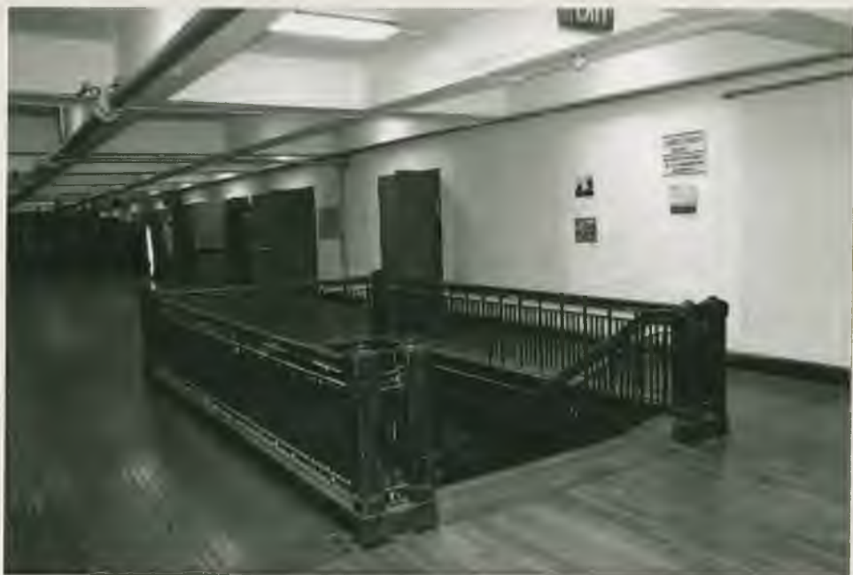
Top landing of staircase, third story (27-9)
