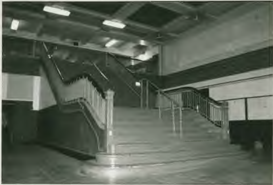
Staircase to second story (27-15)
