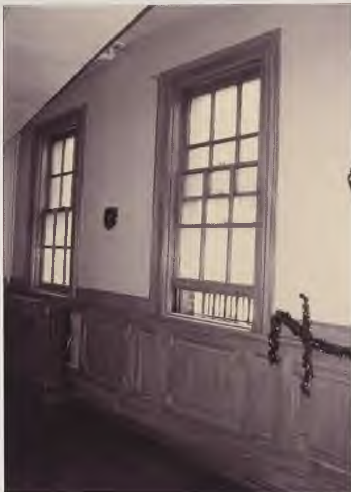
Company meeting room, south end of administration building, first story (27-21)
