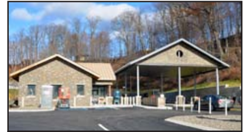
Construction of the new Entry Control Point for the Camp Smith Training Site was completed in 2016.
