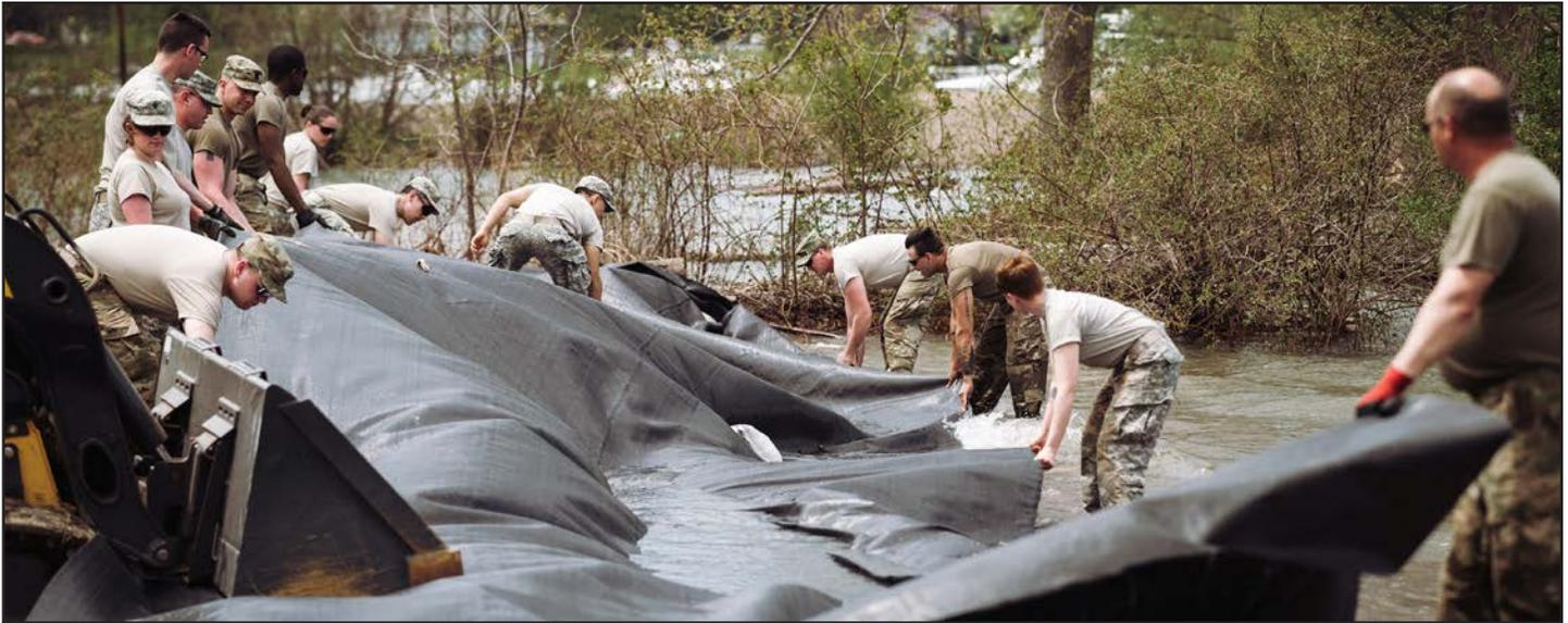
*New York Army National Guard Soldiers setup a tarp, on top of which a barrier is made of stone and sandbags in an attempt to hold off erosion along the Lake Ontario shoreline after rising water levels have resulted in flooding and a state of emergency being declared on May 2 by Gov. Andrew Cuomo, Kendall, N.Y., May 18.*
