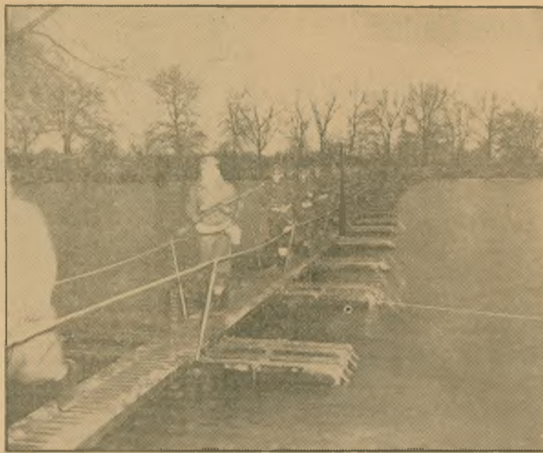
A Company of the 106th Infantry crossing pontoon assault bridge on the run. The Bridge was built across Oxford Lake, South of Anniston by the 102nd Engineers. (Photo by Miller.)
