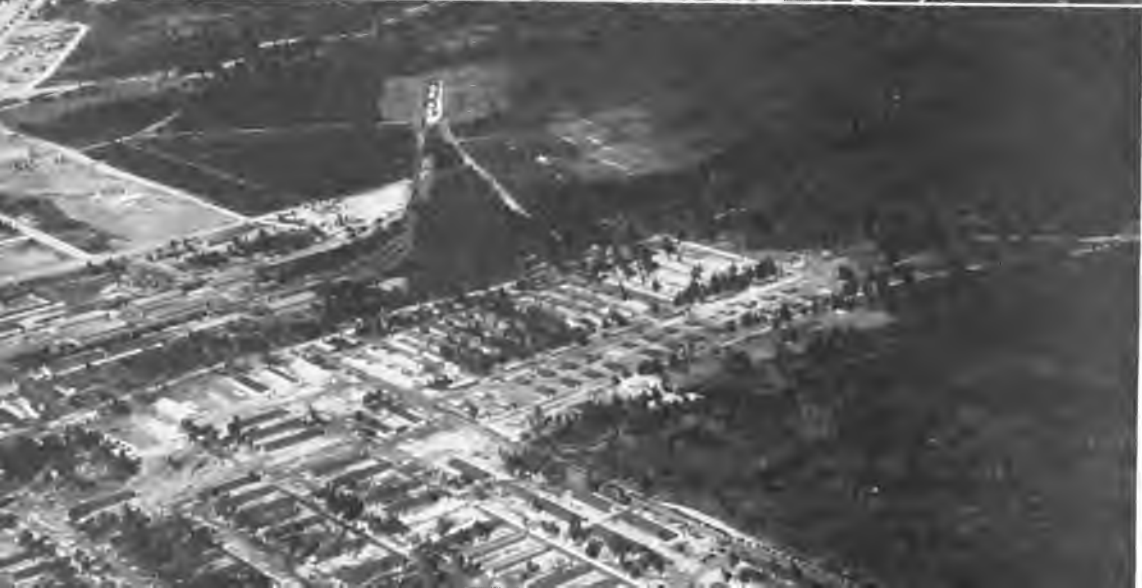
3. New hospital area.
