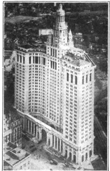
Municipal Building, New York City
