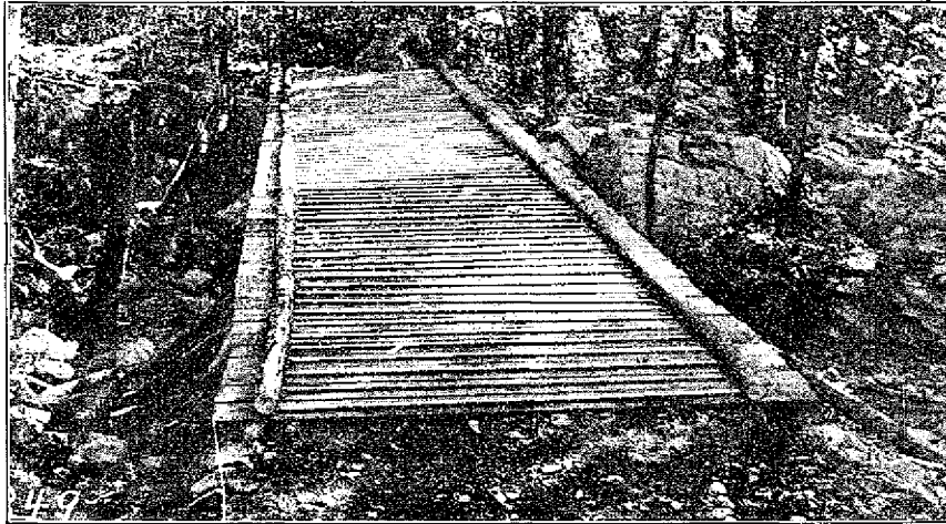
"The Defendum Bridge," Camp Smith, Peekskill, N. Y., the handiwork of the 102nd Engineers.
