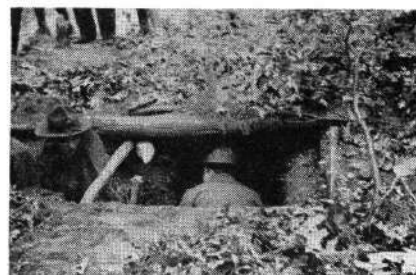
Entering Message Center and telephone switchboard section.
