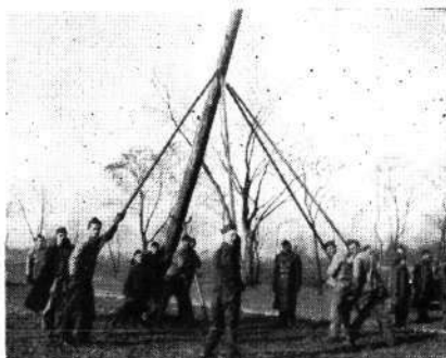
Telephone pole construction.
