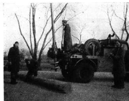
Special gasoline power driven earth boring equipment.
