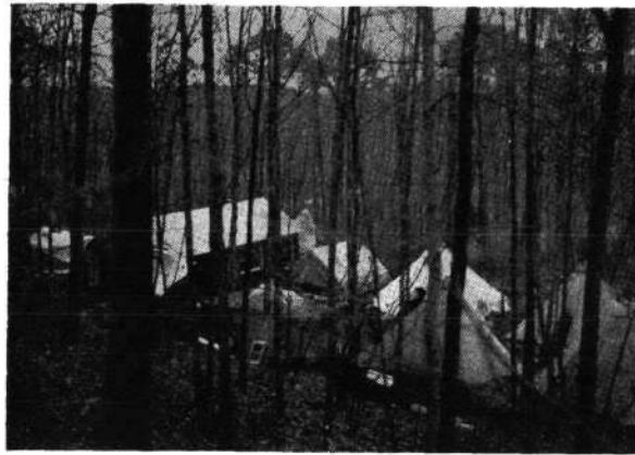
Bottom of page—Progressive Views of Cabin Built by —102d Engineers.
