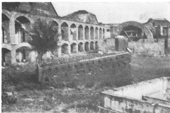
Hot Shot Oven and Ammunition Storage
