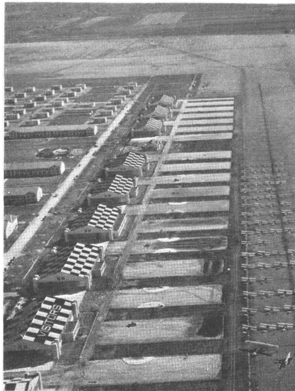
■ A STAGE HANGAR LINE—RANDOLPH FIELD —
