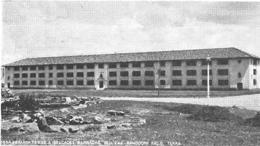
155A-4671-20H-72632-3-13PACADET BARRACKS, BLDG. 243, RANDOLPH FIELD, TEXAS.
