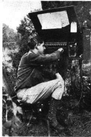
Corp. WM. FEINDEL receiving at the BD11 switchboard
