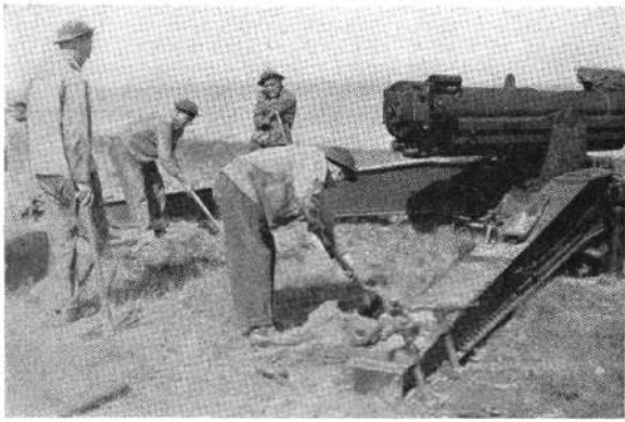
Digging the Recoil Pit
