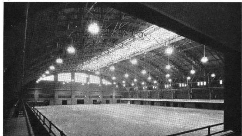
Main Drill Floor
