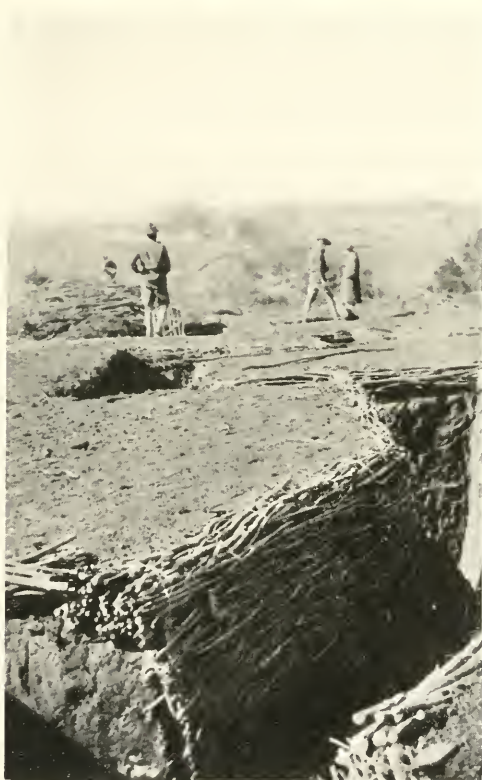
BRUSH REVETMENT—TRENCHES AT CAMP WADSWORTH
