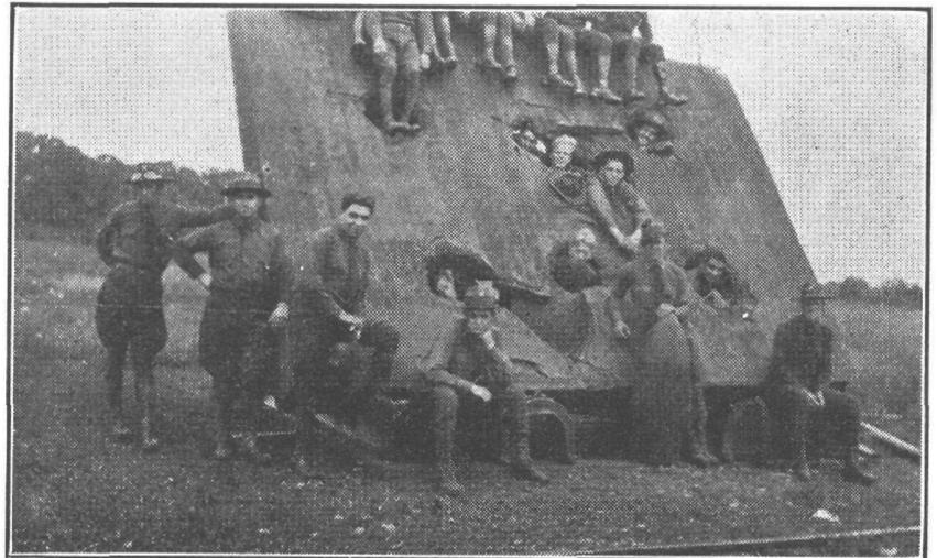
Members of the 102nd Ordnance Co., at Ft. Meade, Md., grouped about an 18" slab of steel which had been penetrated several times by shells fired from a 16" naval gun.
