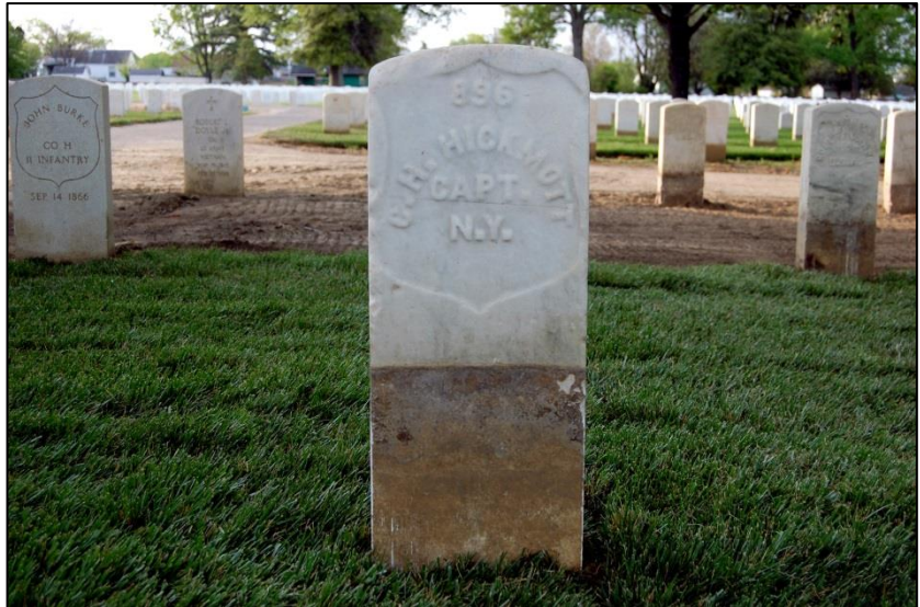
Figure 17: Evidence of stone sinking at Richmond National Cemetery.
